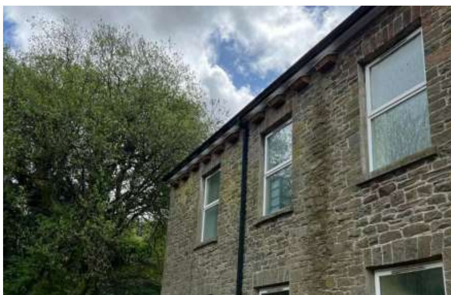
Figure 17. Swift boxes installed on NPTC-owned building in Resolven
